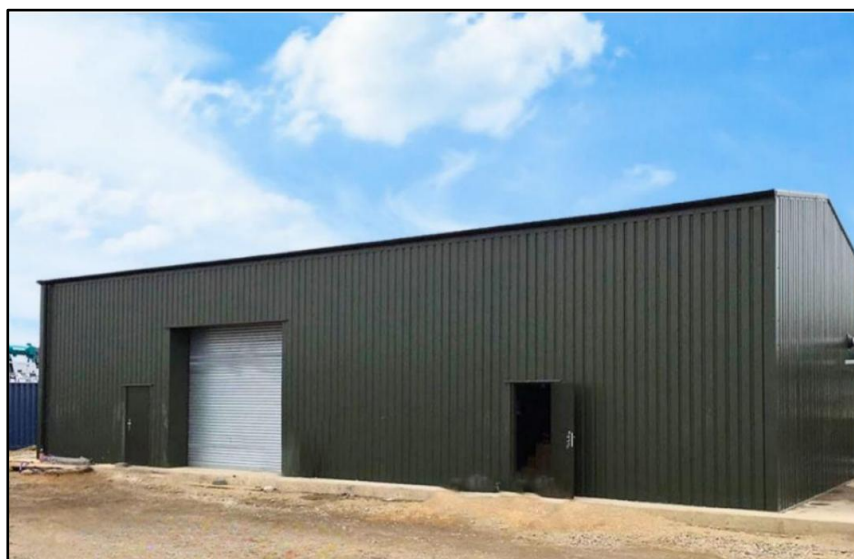
Plate 3.11: Example of a Collector Compound
